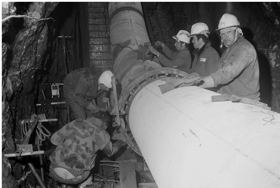
CONSTRUCTION OF A NATURAL GAS PIPELINE IN MEIRINGEN; BRIENZER ROTHORN TUNNEL, SWITZERLAND
