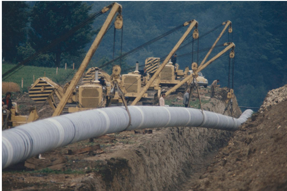
CONSTRUCTION OF A NATURAL GAS PIPELINE IN ROHR, SWITZERLAND
