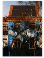
PV INSTALLATION, BREMEN Source: Wikipedia
