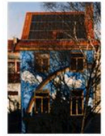
PV INSTALLATION, BREMEN Source: Wikipedia
