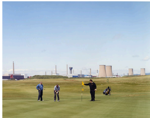
COOLING TOWERS IN THE LANDSCAPE Source: Atlas of Places, Jürgen Nefzger, Fluffy clouds , 2003–2005
