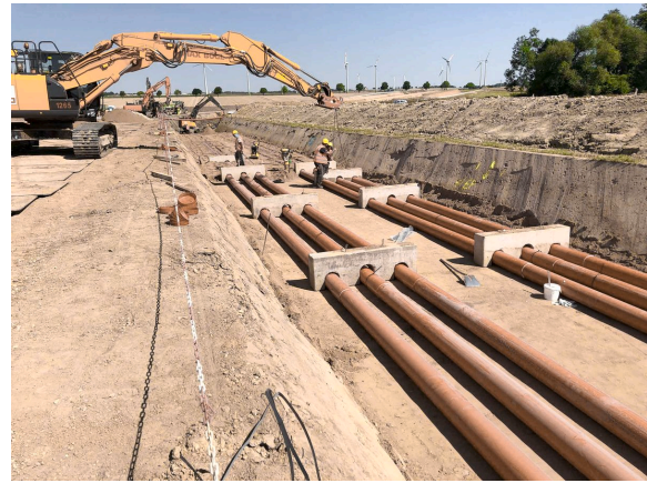
IMPACT ON THE GROUND
