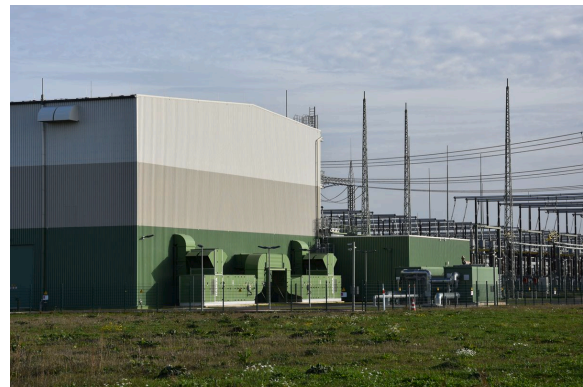
OPERATION BUILDING OF ELECTRICAL SUBSTATION OBERZIER
