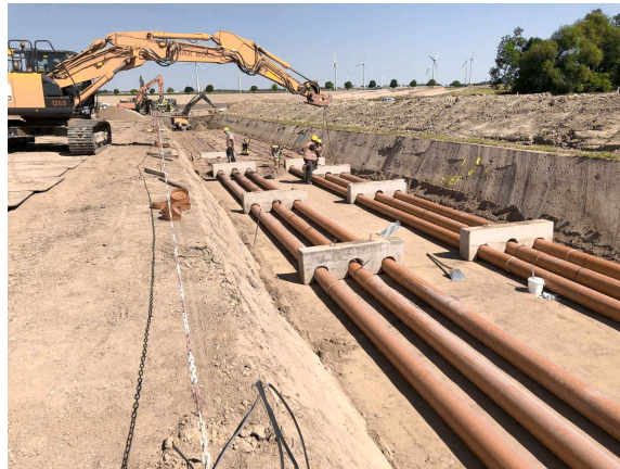
IMPACT ON THE GROUND
