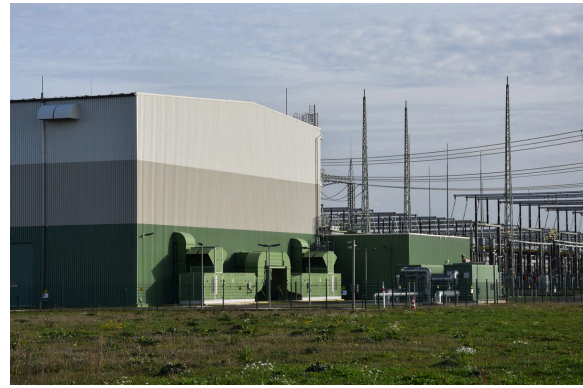
OPERATION BUILDING OF ELECTRICAL SUBSTATION OBERZIER
