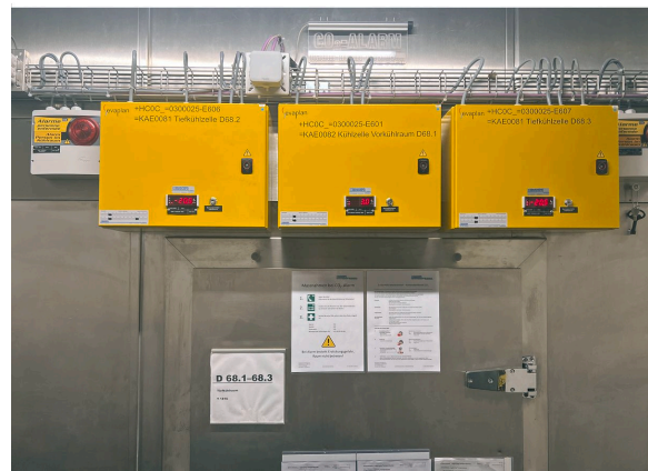
Cold storage regulator at ETH Hönggerberg
