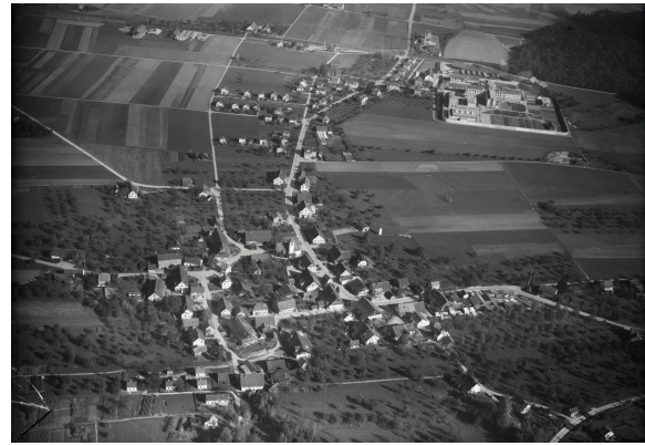
Aerial View of Regensdorf 1948, Source: Friedli Werner, 1948.
