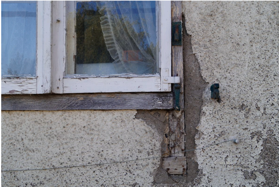
Window frame detail, 2023.
