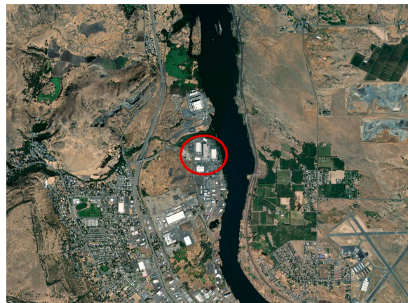
The Dalles data centre is located at the shore of the Columbia River.
