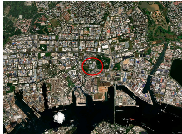
Meta's Singapore data centre is located next to a small river in Singapore.
