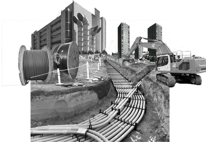
Laying of Fibre Optic Cable. Collage: The Authors.
