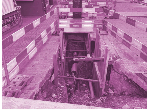
LAYING OF GAS PIPE
