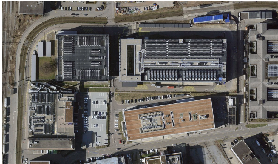
Aerial view of DigitalRealty Campus in Glattbrugg. Photograph: map.geo.admin.ch, 2025.
