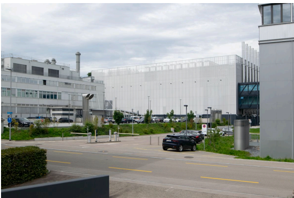
DATA CENTER ZUR 2 DIGITAL REALTY GLATTBRUGG. Photograph: AOT, 2025.
