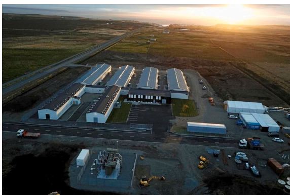
INCONSPICUOUS DATACENTER IN BLÖNDUOS, ICELAND Source: Invest in Iceland, 2023.
