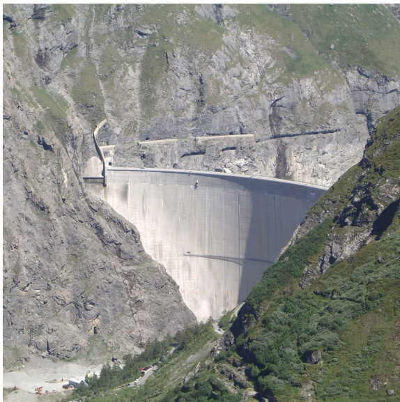
Mavoisin Dam. Source: Source: Olivier Bruchez, 2006.
