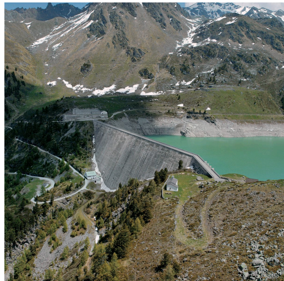
Grande Dixence Dam. Source: Grande Dixence, 2025.
