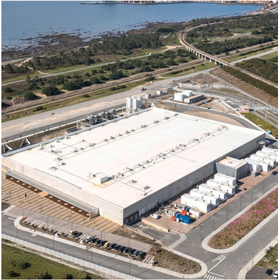
SINES Data Campus. Source: startcampus.pt, 2025.
