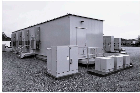
Power transformer. Source: CAT, 2017.
