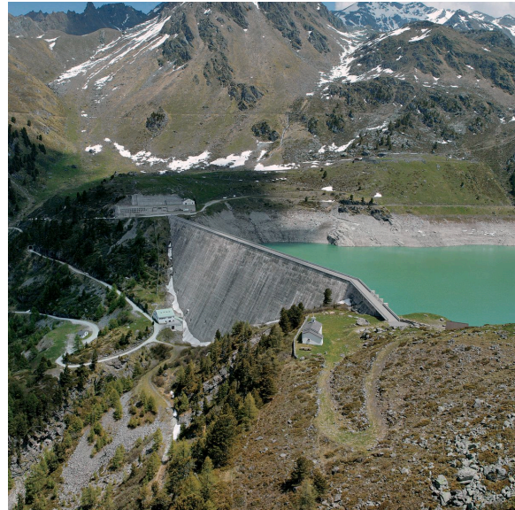
Grande Dixence Dam. Source: Grande Dixence, 2025.
