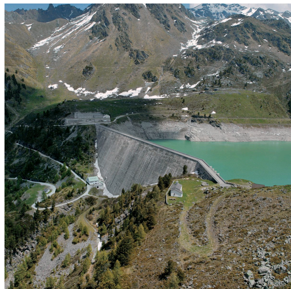
Grande Dixence Dam. Source: Grande Dixence, 2025.
