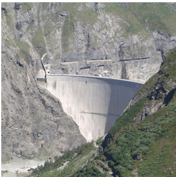
Mavoisin Dam. Source: Source: Olivier Bruchez, 2006.
