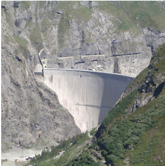
Mavoisin Dam. Source: Source: Olivier Bruchez, 2006.
