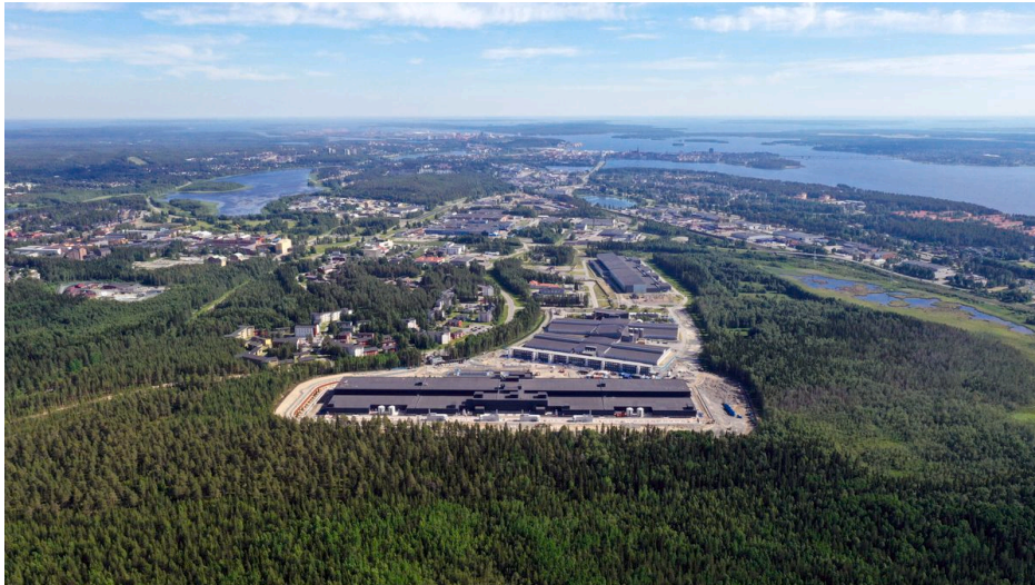
Meta's hyperscale data centre campus in Luleå, Sweden. Source: Sisk, Northern Sweden Data Center, 2026.
