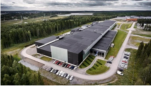
Meta's data centre in Luleå, Sweden. Source: LPI Group, Internal Earthing, 2026.
