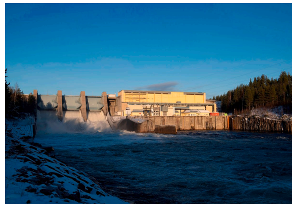
Laxede hydropower plant on the Lule River, Sweden. Source: VekuVaku, 2024.
