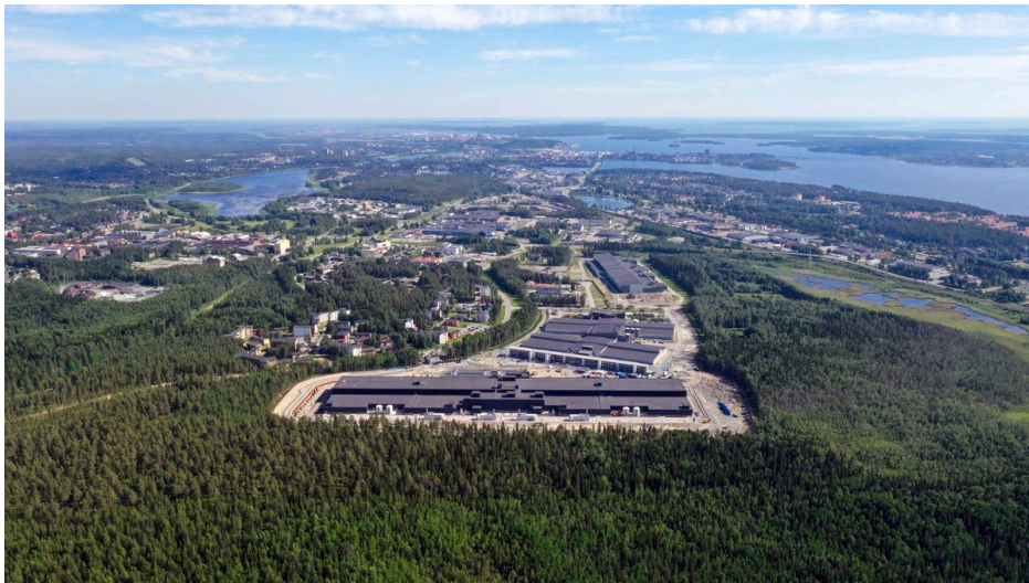
Meta's hyperscale data centre campus in Luleå, Sweden. Source: Sisk, Northern Sweden Data Center, 2026.
