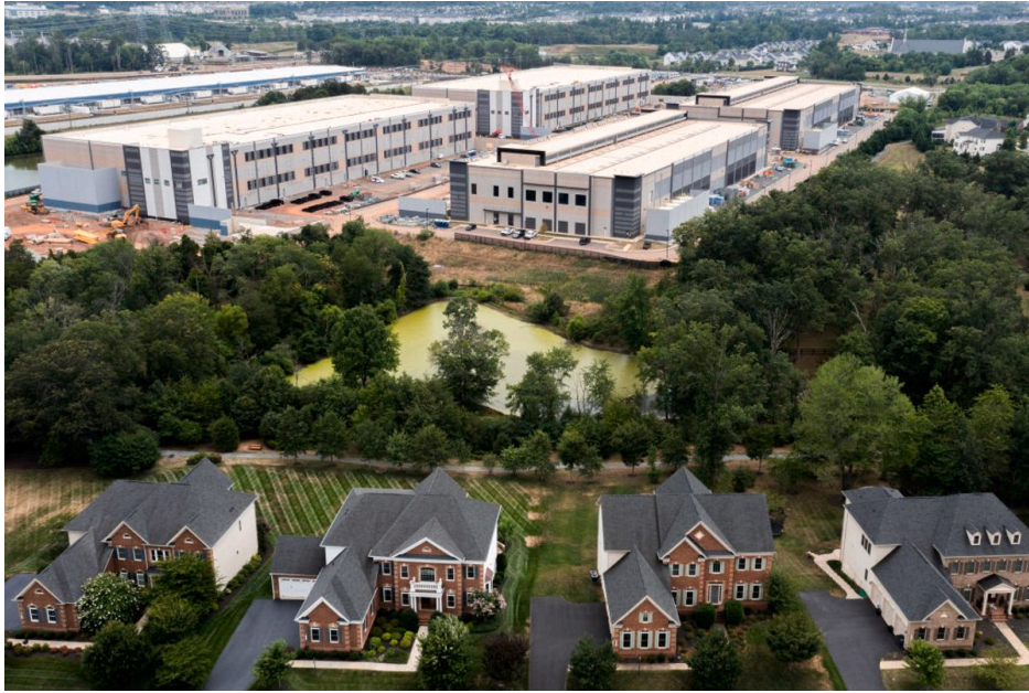
An aerial view shows a data centre situated near single-family homes in Stone Ridge, Va., in 2024. Photograph: Nathan Howard.
