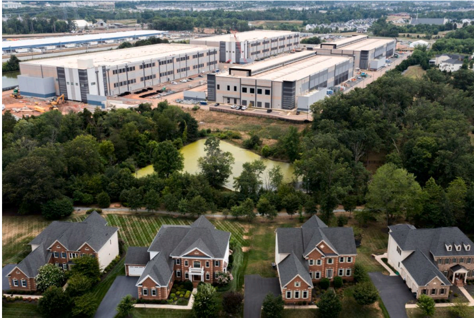
An aerial view shows a data centre situated near single-family homes in Stone Ridge, Va., in 2024. Photograph: Nathan Howard.
