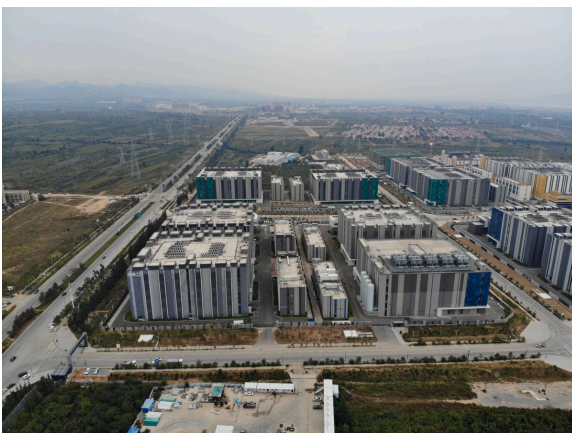
Hoyin Data center in Zhangjiakou, Hebei province, China. Source: Yiqiu Liu, 2024
