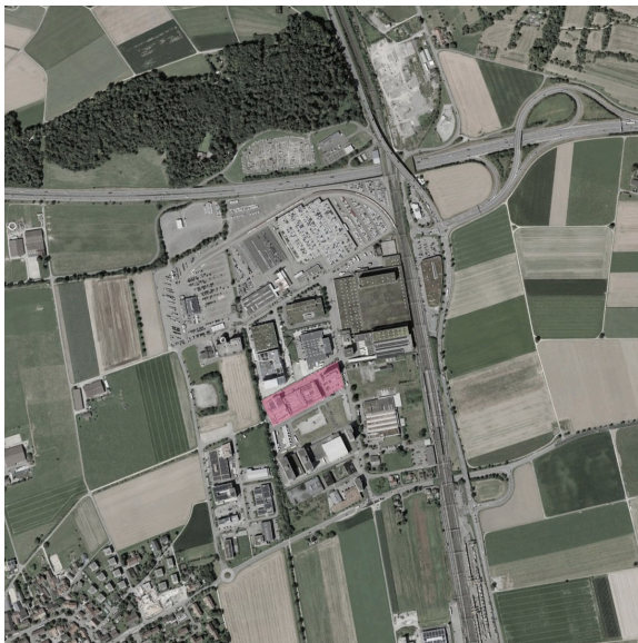
Green data centre Lupfig (Zurich): High-efficiency Swiss data centre with 40 MW IT power, 10,000 m 2 floor area, and capacity for around 80,000 servers.
