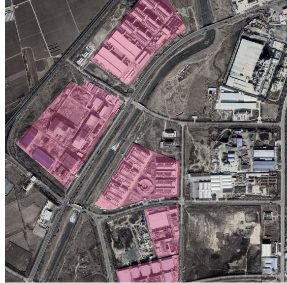
Zhangjiakou data centre cluster: Large-scale regional compute landscape with ~550,000 m 2 data centre area and an estimated capacity of 4.4 million servers distributed across multiple campuses.
