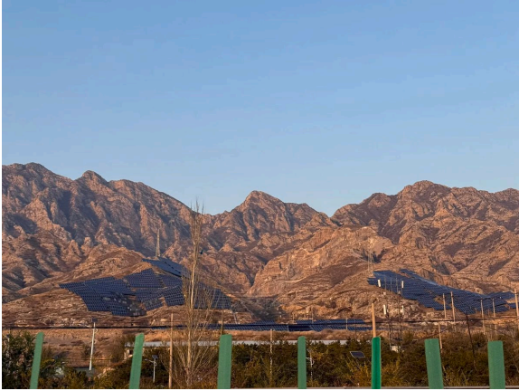
Large-scale solar installations in Zhangjiakou contributing renewable electricity to the region's energy system.
