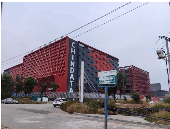
Chindata in Zhangjiakou, Hebei province, China. Source: Yiqiu Liu, 2024
