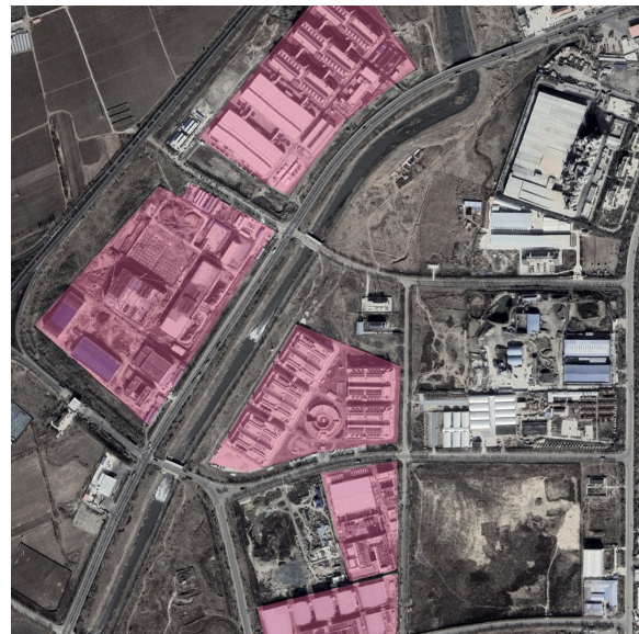
Zhangjiakou data centre cluster: Large-scale regional compute landscape with ~550,000 m 2 data centre area and an estimated capacity of 4.4 million servers distributed across multiple campuses.
