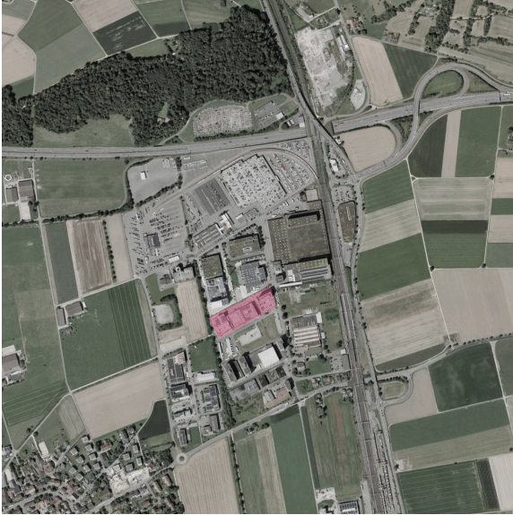
Green data centre Lupfig (Zurich): High-efficiency Swiss data centre with 40 MW IT power, 10,000 m 2 floor area, and capacity for around 80,000 servers.
