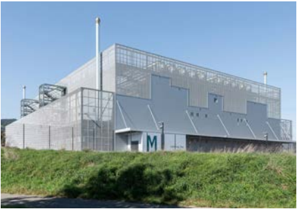
The first of three identical data centres to be built by Green in Dielsdorf. Alone it has a capacity of 30 MW.
