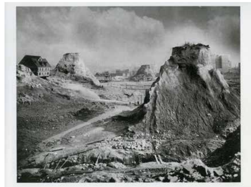
Fig. 6: Ashael Curtis, The Leveling of the Hills to Make Seattle , 1910. Cut-and-Fill: The basic earthworks technique used to realize a buildable urban plane consists in breaking hills and dumping them into the sea, swamps or other low-lying areas.
