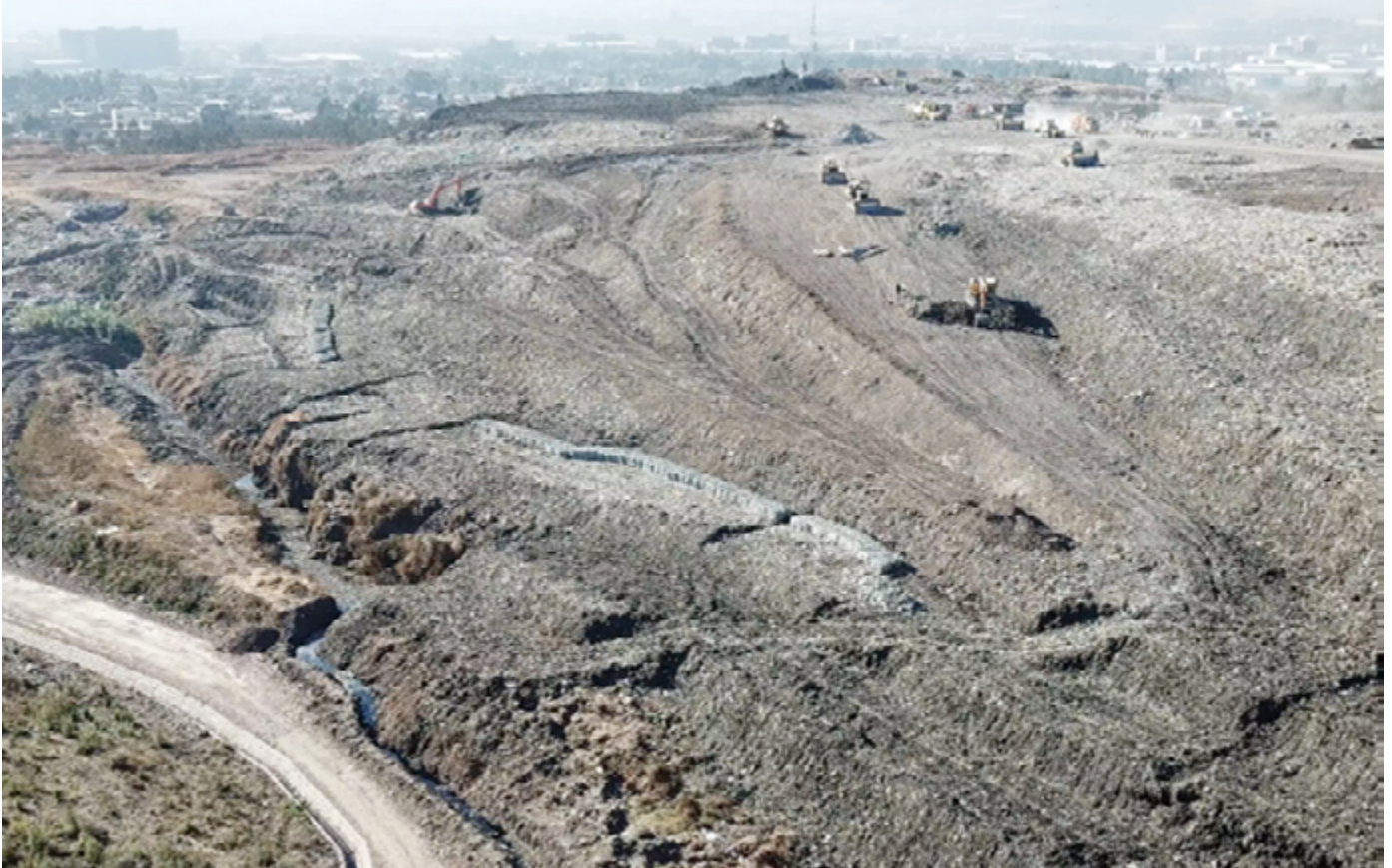
Reppie/Koshe dumpsite emergency rehabilitation project
