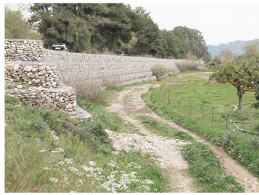
Flooding Protection Wall
