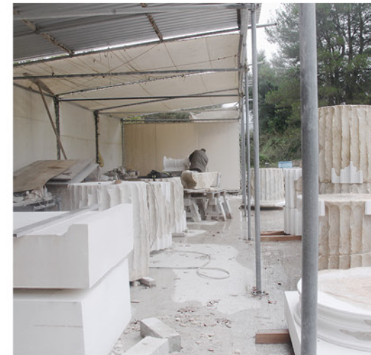
The stone masons' working place and storage on site, 2016
