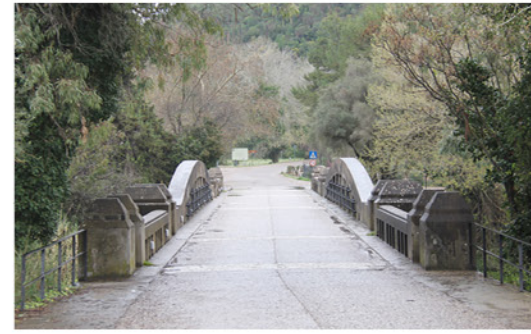
5 The bridge over the Kladeos river
