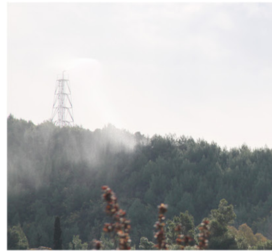
7 A fire protection tower
