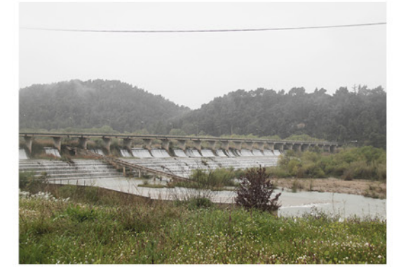
17 The dam of Alfeios River
