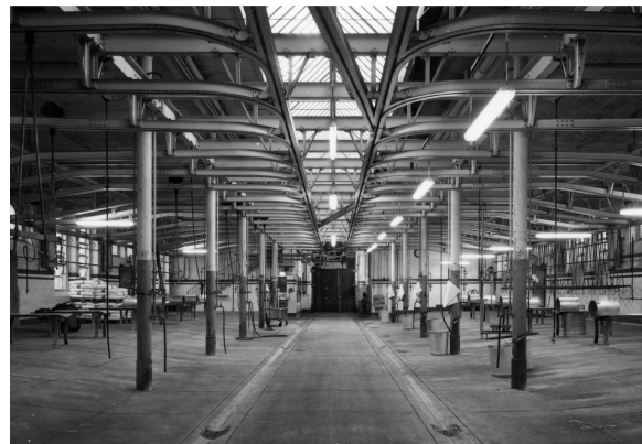
1980: empty slaughter hall for small cattle with numerous slaughtering stations, slaughterhouse Zurich. Source: Baugeschichtliches Archiv der Stadt Zürich.
