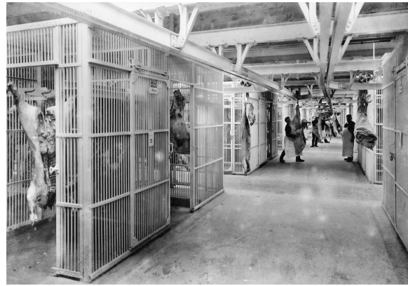
1909: slaughter bodies moved by butchers in the cold storage, slaughterhouse Zurich. Photograph: Heinrich Wolf-Bender. Source: Baugeschichtliches Archiv der Stadt Zürich.
