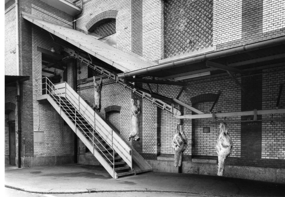
1960: slaughter bodies carried over stairs to the exterior by the transport rail, slaughterhouse Zurich. Photographer: Erwin Kuenzi. Source: Baugeschichtliches Archiv der Stadt Zürich.
