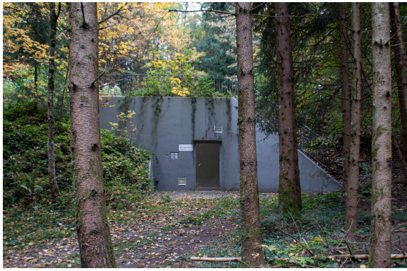
Disguised water infrastructure.
