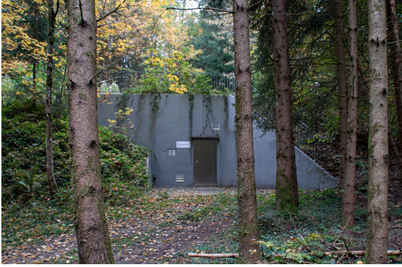
Disguised water infrastructure.
