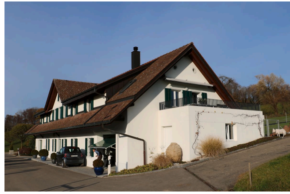
Residential house, former cheese dairy.
