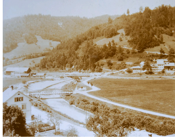
Töss Correction under Construction
