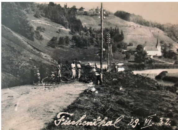
Road Construction Fischenthal 1932
