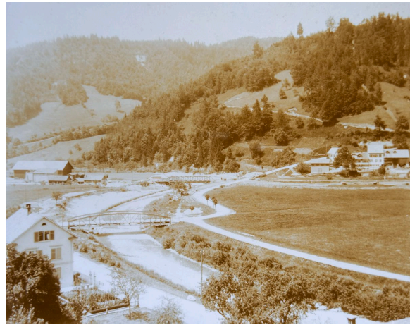
Töss Correction under Construction
