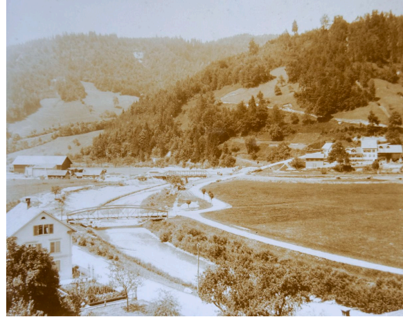
Töss Correction under Construction
