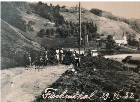
Road Construction Fischenthal 1932
