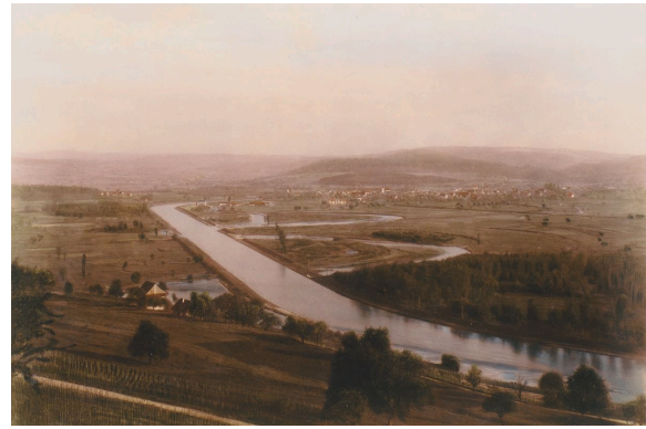
The river course at the Grien-Inseln after the correction. Photograph: Ortsmuseum Dietikon, 1895.
