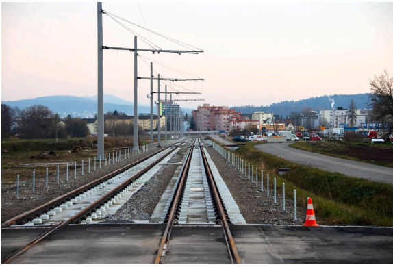
Limmattalbahnhof tracks towards Dietikon. Photograph: Jonas Schmid, 2021.
