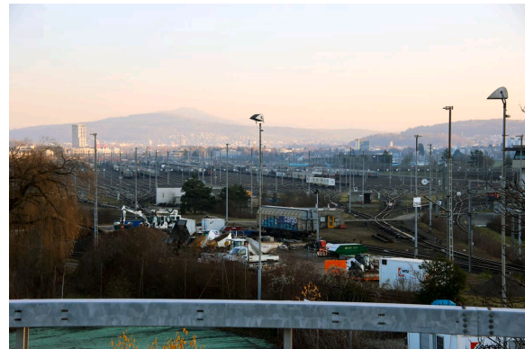
View over the marshalling yard. Photograph: Jonas Schmid, 2021.
