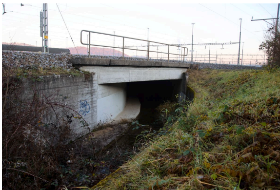
Canalization of Dorfbach under marshalling yard. Photograph: Jonas Schmid, 2021.
