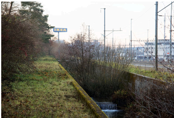
Canalization of Dorfbach near Kreuzäcker. Photograph: Jonas Schmid, 2021.
