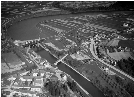
View on the reservoir of the power station in Wettingen. Photograph: Werner Friedli, 1939.
