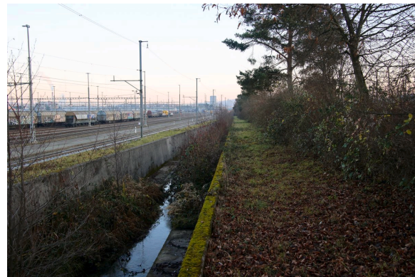
Canalization of Dorfbach at marshalling yard. Photograph: Jonas Schmid, 2021.
