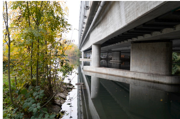
Crossing of the highway bridge over the Limmat. Photograph: Florian Hofmann, 2021.
