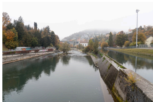
Canalized river course. Photograph: Florian Hofmann, 2021.
