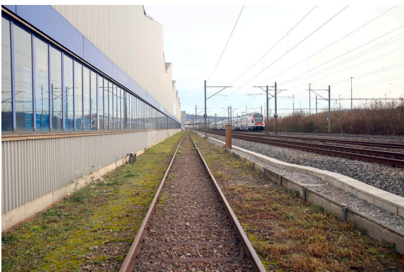
Unused railway between Silbern and the marshalling yard. Photograph: Jonas Schmid, 2021.
