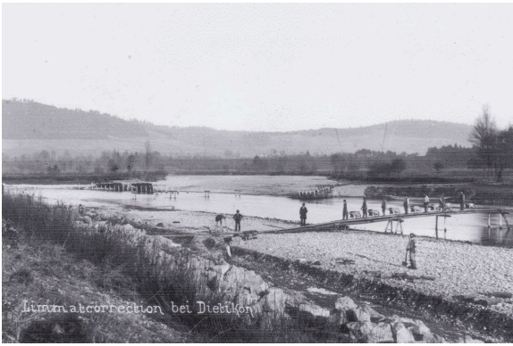
Construction work on the Limmat correction. Photograph: Ortsmuseum Dietikon, approx 1890.
