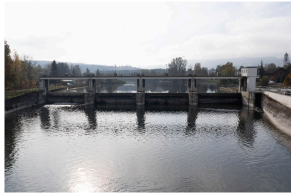
Dam next to Dietikon. Photograph: Florian Hofmann, 2021.
