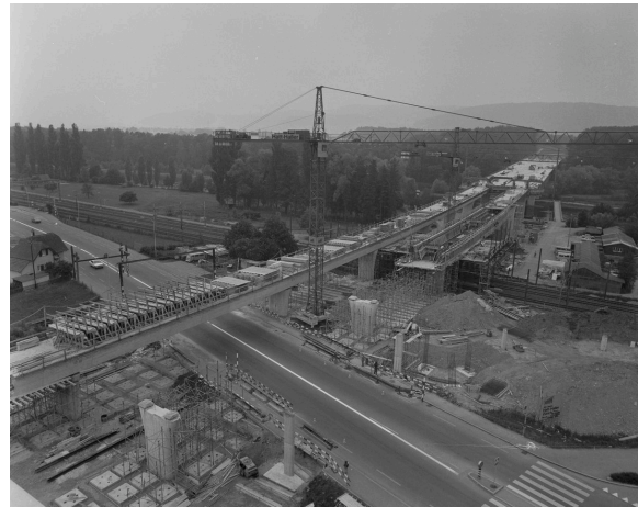
Construction of the highway bridge in Glanzenberg. Photograph: Patrick Lüthy, 1983.
