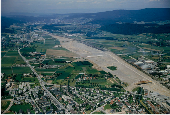
View on the construction of the marshaling yard. Photograph: Comet Photo AG, 1974.
