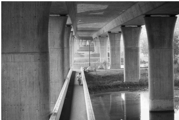
Highway bridge over the Limmat in Glanzenberg. Photograph: Heinz Baumann, 1985.
