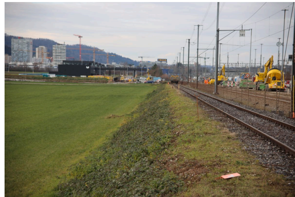
Railtrack Kreuzäcker area. Photograph: Jonas Schmid, 2021.
