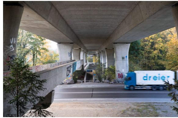
Glanzenberg highway bridge over Limmat. Photograph: Florian Hofmann, 2021.
