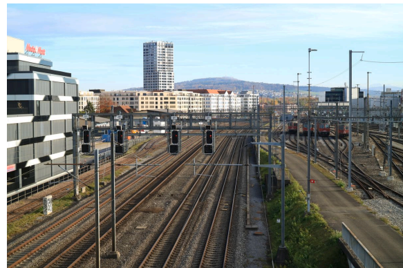
Southeastern end of the marshaling yard in Dietikon. Photograph: Markus Nyfeler, 2021.
