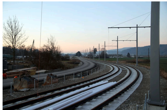
Limmattalbahn tracks. Photograph: Jonas Schmid, 2021.
