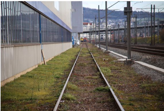
Railtrack Silber area. Photograph: Jonas Schmid, 2021.
