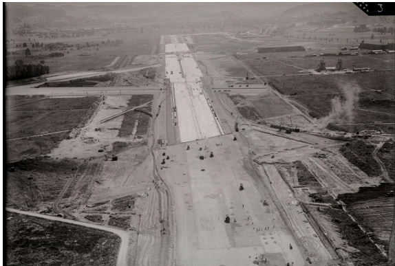
Runway construction for the new Zurich airport. Source: ETH Library - Bildarchiv, 1947.
