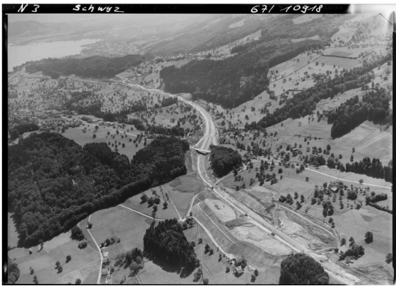
1960: Construction of the A3 motorway from Zurich to Pfäffikon. Source: e-pics. [https://ba.e-pics.ethz.ch/catalog/ETHBIB.Bildarchiv/r/104164/viewmode=infoview/qsr=A3%20bei%20Pfäffikon]
