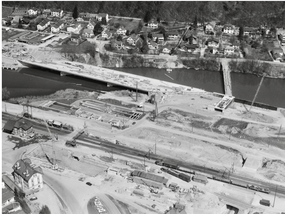
Construction of the Highway A1 in 1969. Source: ETH Bildarchiv.
