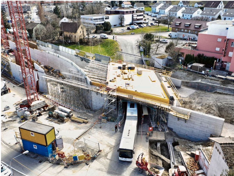
Limmattalbahn, construction finishes in Winter 2022. Source: ACS Partner
