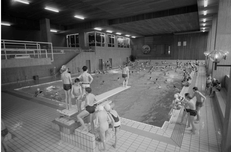
A swimming pool - Still existing. Source: ETH Bildarchiv, Heinz Baumann, 1974.
