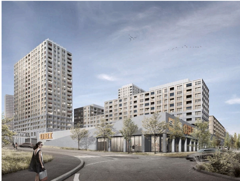
Tivoli Garten, construction finishes in Summer 2024. Source: feldmann-Bau.ch
