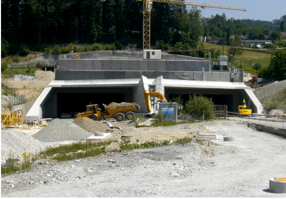
Construction Aeschertunnel in 2009. Source: wikipedia.org
