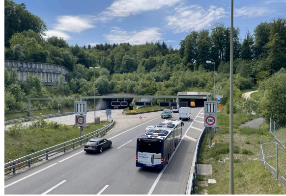
Aeschertunnel east side.
