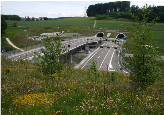
Aeschertunnel west side. Source: wikipedia.org
