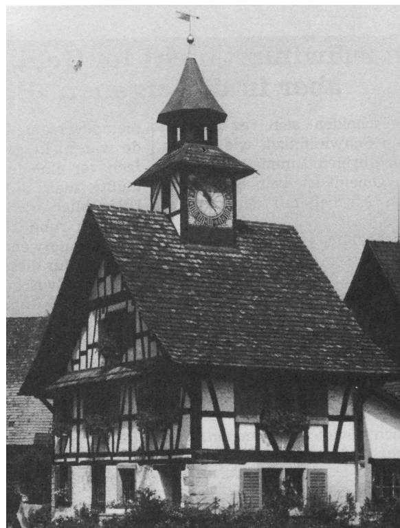
Türmlihaus after restoration. Source: E. Gugerli, "Dokumentation Aesch", Band 1-3, 1983.
