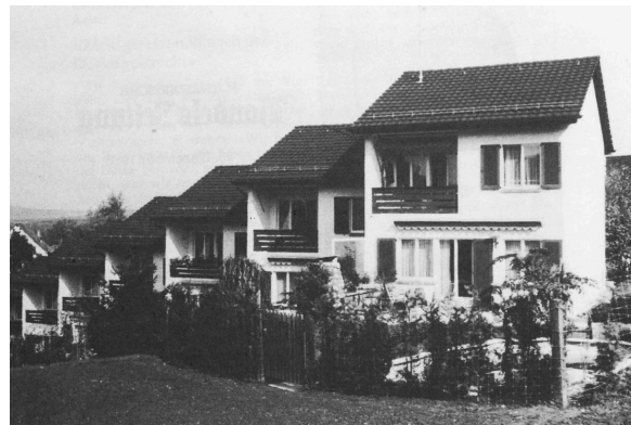
Construction of serial housing. Source: E. Gugerli, "Dokumentation Aesch", Band 2, 1983.
