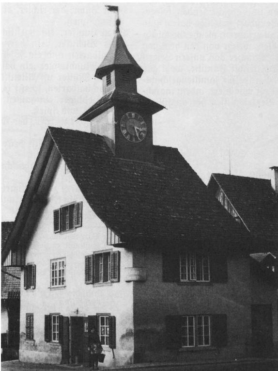
Türmlihaus before restoration. Source: E. Gugerli, "Dokumentation Aesch", Band 1-3, 1983.
