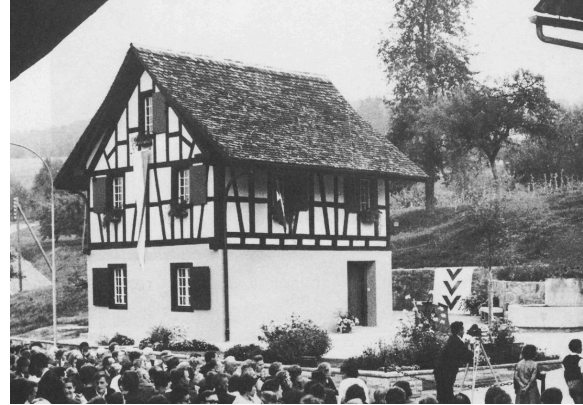
Dorfmuseum after restoration. Source: E. Gugerli, "Dokumentation Aesch", Band 1-3, 1983.
