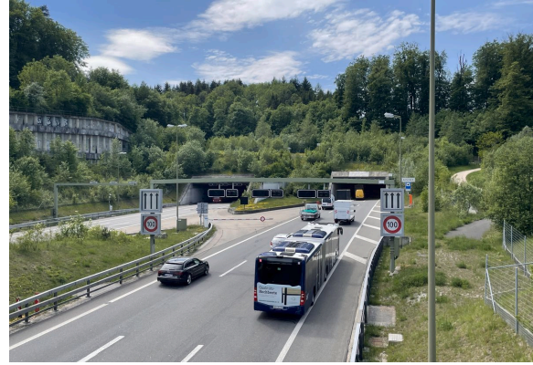
Aeschertunnel east side.
