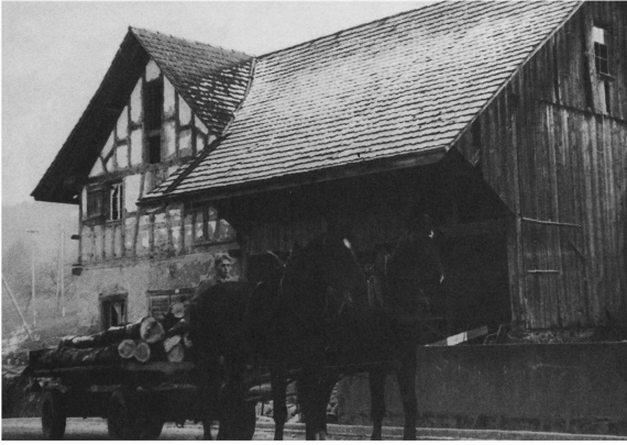
Dorfmuseum before restoration. Source: E. Gugerli, "Dokumentation Aesch", Band 1-3, 1983.
