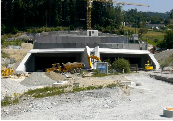
Construction Aeschertunnel in 2009. Source: wikipedia.org
