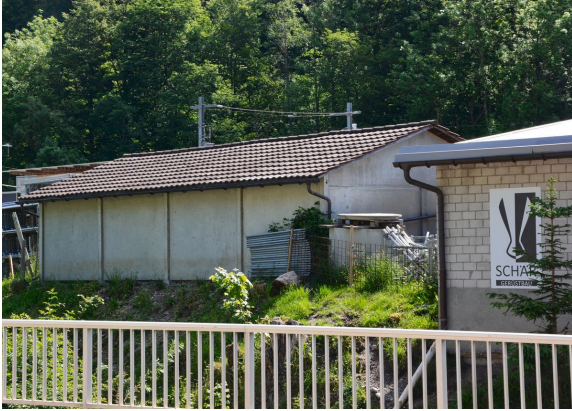
Around the train station there are businesses such as scaffolders who need more space...
