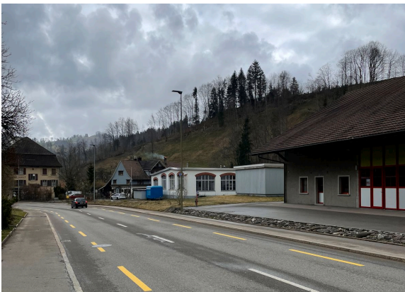
Firefighter's headquarters follow reused factory buildings.
