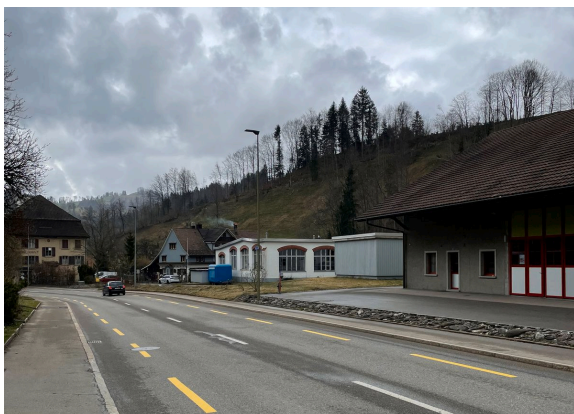
Firefighter's headquarters follow reused factory buildings.
