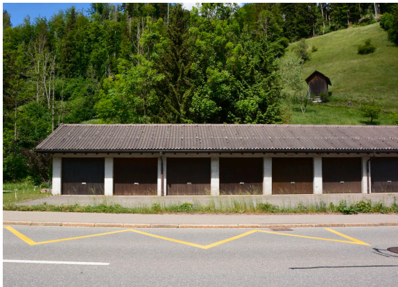
The bus stop operates from 20:30 - the train is only scheduled until dinner.
