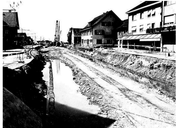
Undertunneling of the Forchbahn, 1977. Source: Forchbahn renovation. [ https://docplayer.org/166849505-Tunnel-zumikon-sanierung.html ]
