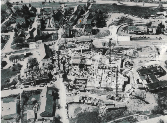
Village square building site, 1975. Source: Wohnort: 8126 Zumikon, 2009.
