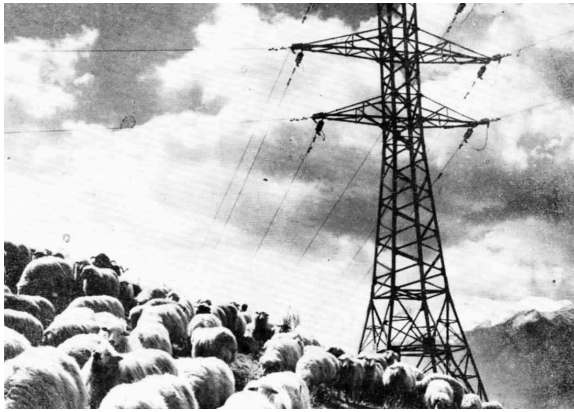
The electrification of the country is fully completed in Albania on October 25th, 1970. Source: Albania Today , No. 3, May/June 1973.
