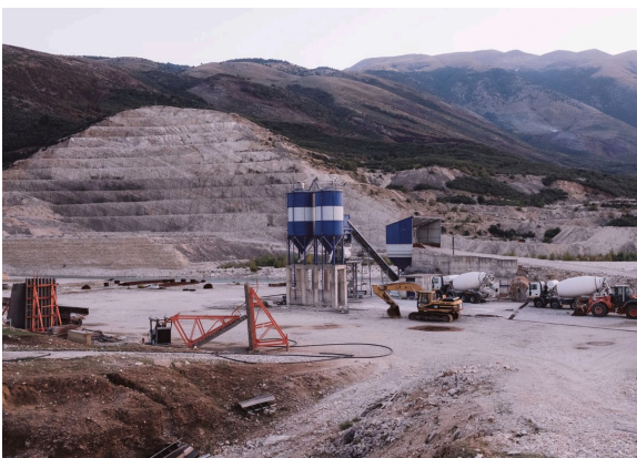
Hydropower construction site Kalivaç. Photographer: Nick St. Oegger [ http://www.stoeggerphotography.com/ ].
