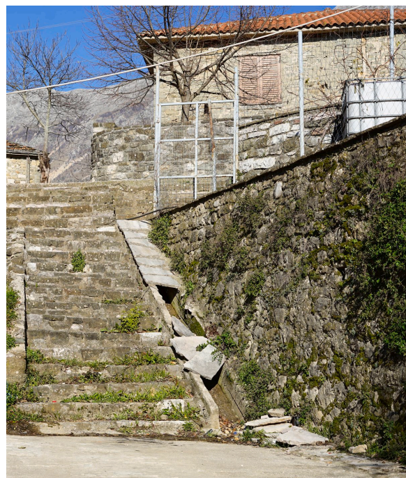
Dysfunctional water channel in Dhoksat. Photographer: Gyler Mydyti.
