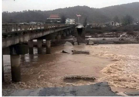
Collapsed bridge between in Dropull near Gjirokastër after heavy rainfalls in December 2017. Source: Periskopi [<https://www.periskopi.com/permytjet-neshqiperi-shemben-pese-ura-ne-gjirokaster/>].
