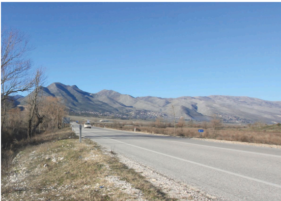
Primary road. Photograph: Nazlı Tümerdem.
