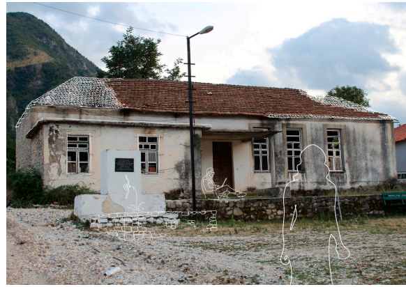
Perspective of the Prongji workshop in an abandoned school. Photograph: Gyler Mydyti, 2019.
