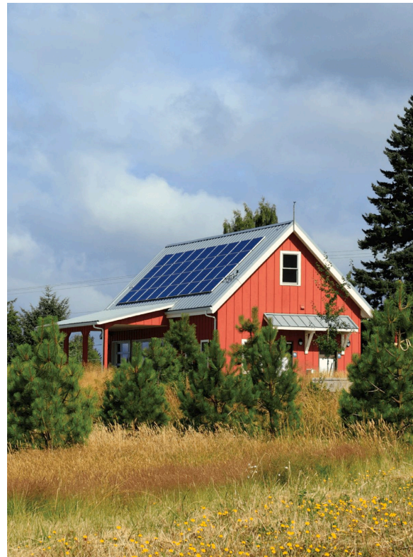
IMAGE OF PHOTOVOLTAIC ON ROOF ONLY.
