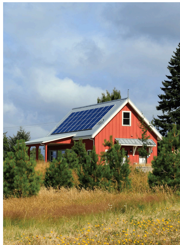
IMAGE OF PHOTOVOLTAIC ON ROOF ONLY.
