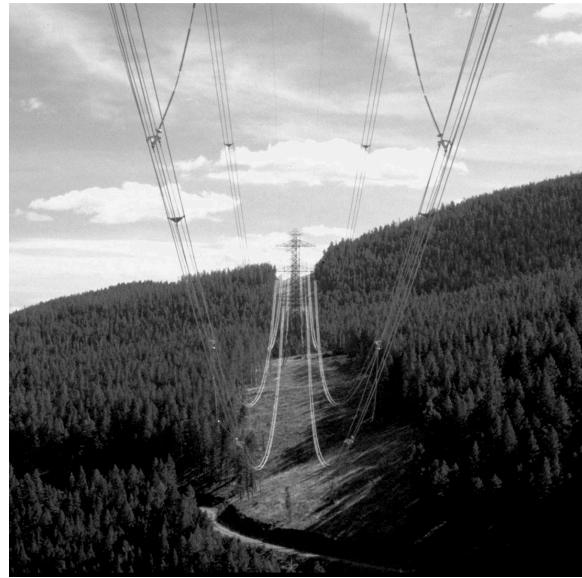
HIGH VOLTAGE POWER LINE LEAVING ITS TRACES IN THE LANDSCAPE.
