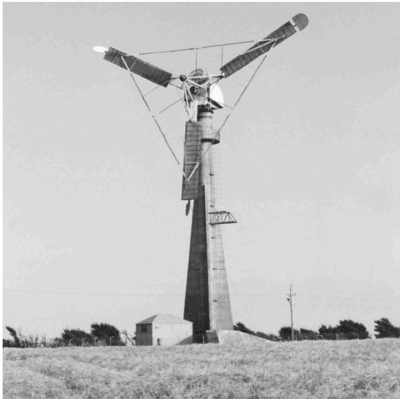
DANISH GEDSER-PLANT IN 1957—ONE OF THE INNUMERABLE WIND TURBINE PROTOTYPES.
