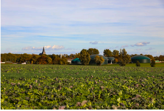
PAEFFGEN BIOGAS PLANT
