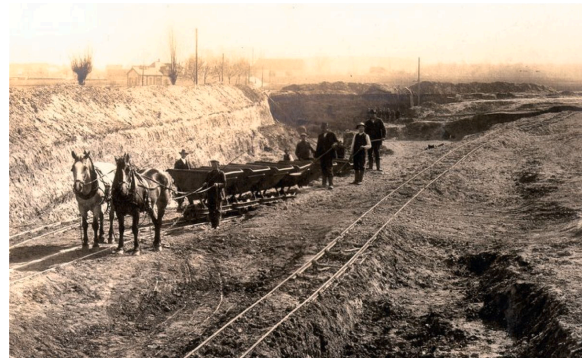
BROWN COAL TRANSPORTATION WITH HORSE-DRAWN LORRIES BEFORE RAILWAYS WERE ESTABLISHED Photograph: LMBV-Archiv, 1912.
