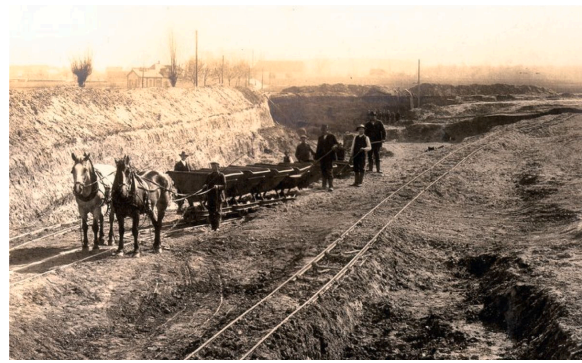
BROWN COAL TRANSPORTATION WITH HORSE-DRAWN LORRIES BEFORE RAILWAYS WERE ESTABLISHED Photograph: LMBV-Archiv, 1912.
