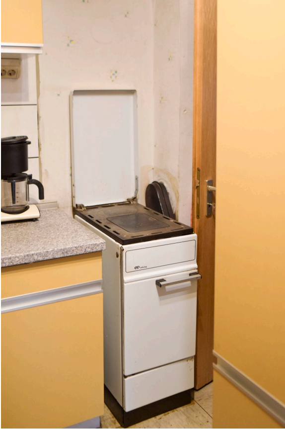
The coal stove in the kitchen.
