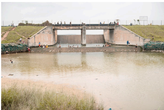
DAM AT THE MUKA KUNING RESERVOIR IN BATAM, INDONESIA.
