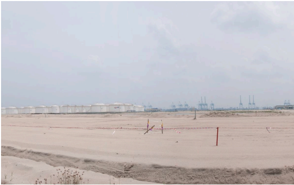
AN OIL TERMINAL BUILT ON RECLAIMED LAND. ATB, TANJUNG BIN, MALAYSIA.
