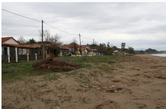
ALONG THE LOCAL COAST: ILLEGAL VACATION HOMES.
