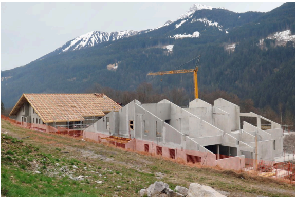
Construction project in the valley.
