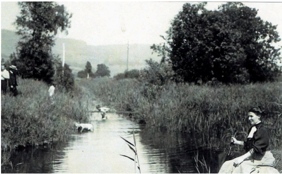
Swimming at the Dürrengraben in 1918. Source: otelfingen-ansichtskarten.ch, 2023
