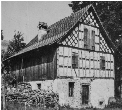
Former communal dairy in Hirzel-Siten. Undated photograph, ca. 1920s. Source: Winkler, Jürg, Der Hirzel. Bild einer Gemeinde . Hirzel: Jürg Winkler, 1989.
