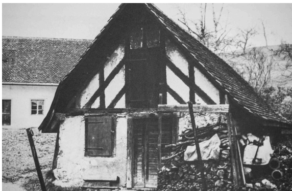
FORMER COMMUNAL DAIRY IN HIRZEL-KIRCHE. UNDATED PHOTO, APPROXIMATELY 1920S. Source: Winkler, Jürg, Der Hirzel. Bild einer Gemeinde . Hirzel: Jürg Winkler, 1989.
