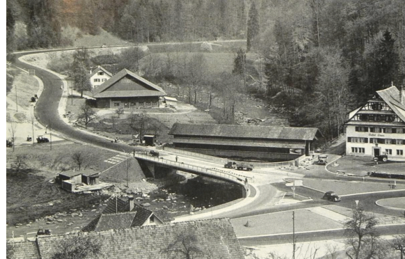
OLD "BABENWAG" BRIDGE, WHICH CARRIED THE MULE TRAIL, BEING REPLACED BY THE NEW HIRZEL PASS, 22 MAY 1960.
