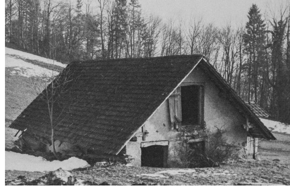
Former communal dairy in Hirzel-Chalbisau, built in the 18th century. Undated photograph, ca. 1900s. Source: Renfer, Christian, Die Bauernhäuser des Kantons Zürich. Band 9-11 . Basel: Schweizerische Gesellschaft für Volkskunde, 1982.
