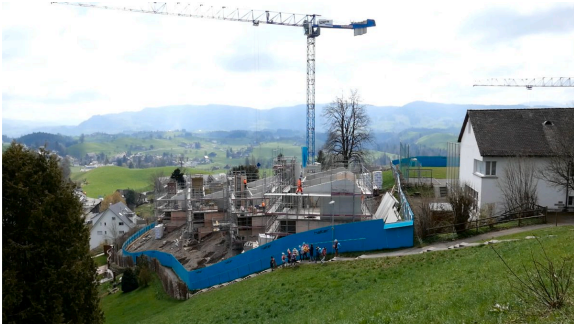
CONSTRUCTION SITE IN THE CENTRE OF THE VILLAGE. Photograph: By the authors.
