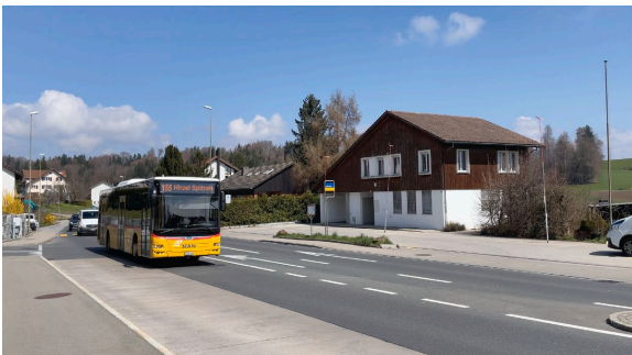
THE ABANDONED POST OFFICE ALONG THE MAIN ROAD, THE HIRZEL PASS. Photograph: By the authors.
