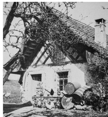
Former communal dairy in Hirzel-Rothus. Undated photograph, ca. 1960s. Source: Winkler, Jürg, Der Hirzel. Bild einer Gemeinde . Hirzel: Jürg Winkler, 1989.
