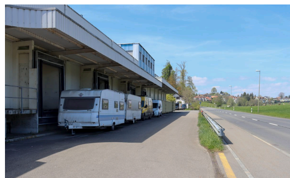
TODAYS ABANDONED HIRZ FACTORY. Photograph: Leon Bloch.
