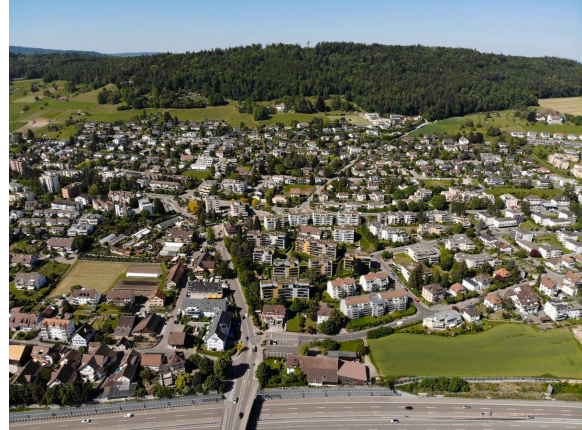
ARIAL VIEW 2022. Source: Gemeinde Unterengstringen [ https://www.unterengstringen.ch ], 2023.
