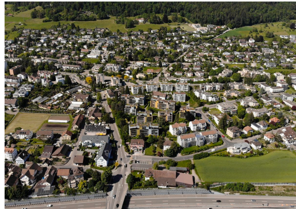
ARIAL VIEW 2022. Source: Gemeinde Unterengstringen [ https://www.unterengstringen.ch ], 2023.
