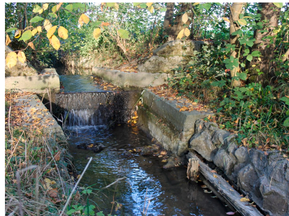
Canalised Chatzenbach. Source: Jan Aebi, 2023.
