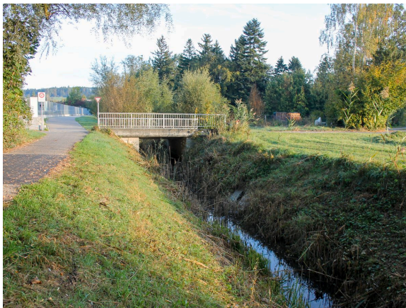
Canalised Chatzenbach. Source: Jan Aebi, 2023.
