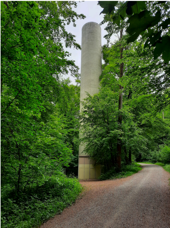
Chimney at Strickhofstrasse 101, Irchel Campus. Source: Own Picture, 2024.
