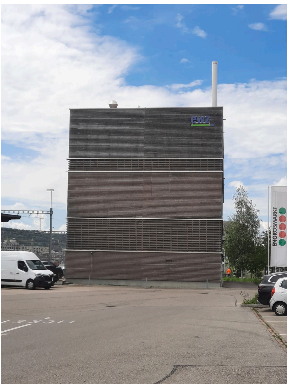
Energy Centre at Aargauerstrasse. Source: Own Picture, 2024
