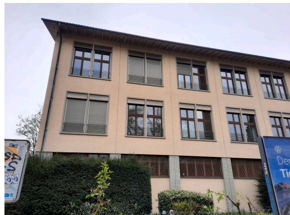
Data Centre Equinix at Letzigraben 75. Source: Own Picture, 2024.
