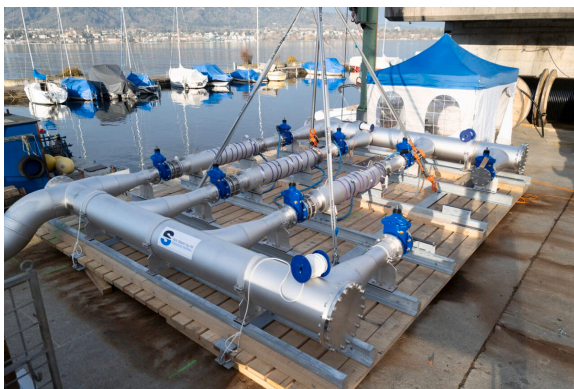
Pipes In the Lake. Source: powernewz.ch, 2022. [ https://www.powernewz.ch/rubriken/waerme-und-kaelteversorgung/seewasserverbund-bahnhofstrasse/ ]
