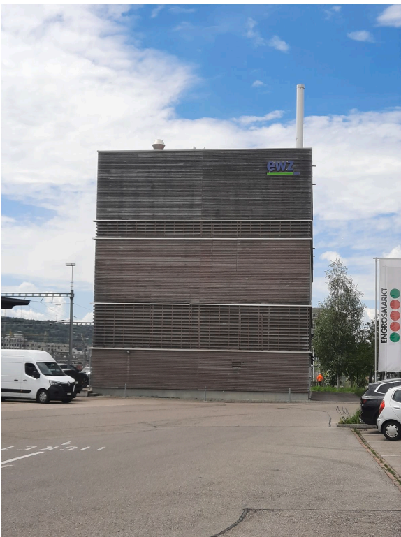
Energy Centre at Aargauerstrasse. Source: Own Picture, 2024
