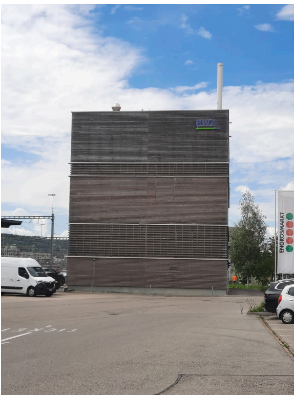
Energy Centre at Aargauerstrasse. Source: Own Picture, 2024
