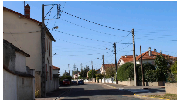
Actual Street in France with above ground Electricity Cables. Source: Jean-François Vaizand, Mesinfos.
