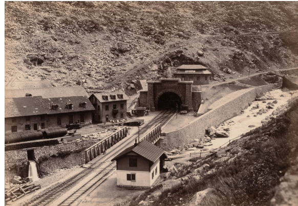
Entrance Göschenen around 1889 Source: Wikipedia, Gotthardtunnel
