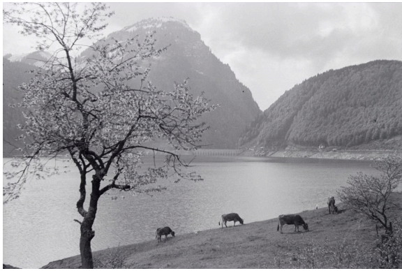
Picture of the village Innerthal after it was demolished. Source: Walter Mittelholzer, 1937.
